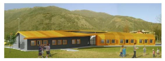
The "type" section of the building is with two slopes, never equal to itself, covers the two parts to intersect at the highest point in the atrium that corresponds to the space able to "capture" the natural light and distribute it along two corridors. A large skylight attenuates the sunlight of summer and welcomes the lowest winter.
